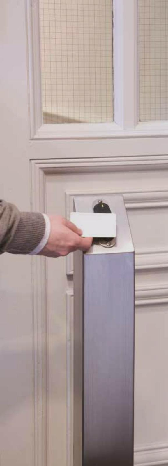
It is possible to eliminate the need for physical contact with ironmongery through the specification of access control, particularly with regards to the activation of the electronic lock.
