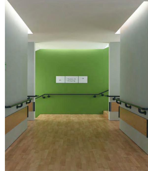
Example of handrails with good visual contrast
