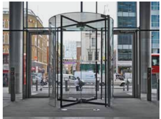
Power operated revolving door
