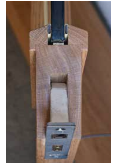
Intumescent around lock
