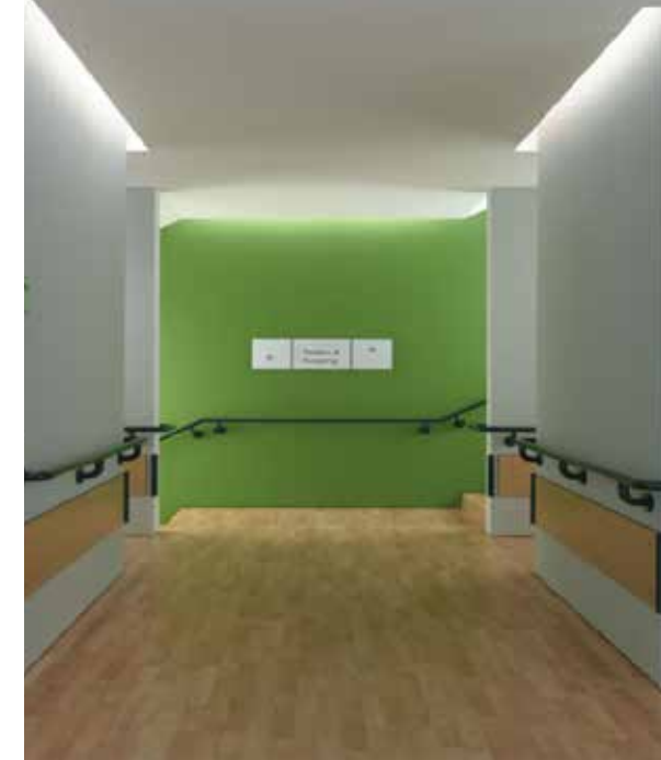
Example of handrails with good visual contrast
